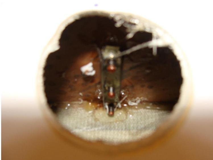
Assembly is relatively simple. The main concern is lack of space. The racks are glued to the wooden beam so they cannot work loose again. This makes it possible to replace or re-tightening the bolts later.
